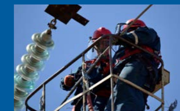
Akhtubinskaya solar power plant with
